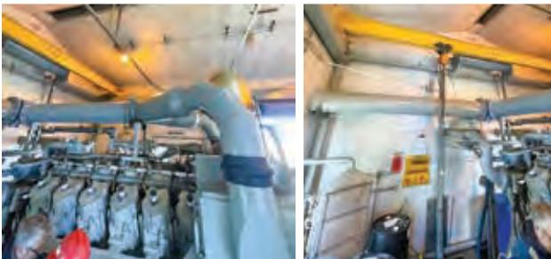
New larger intake piping with diverter
