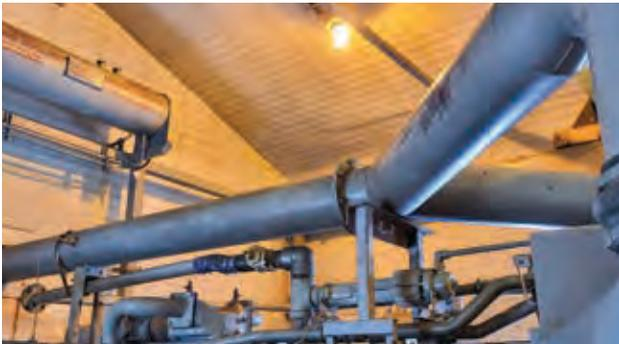
Old undersized intake without air mixture/diverter
