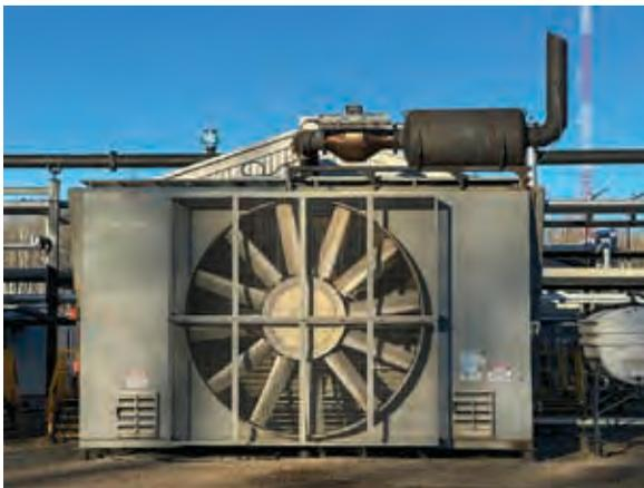
Muffler shortened to allow installation of catalytic converter
